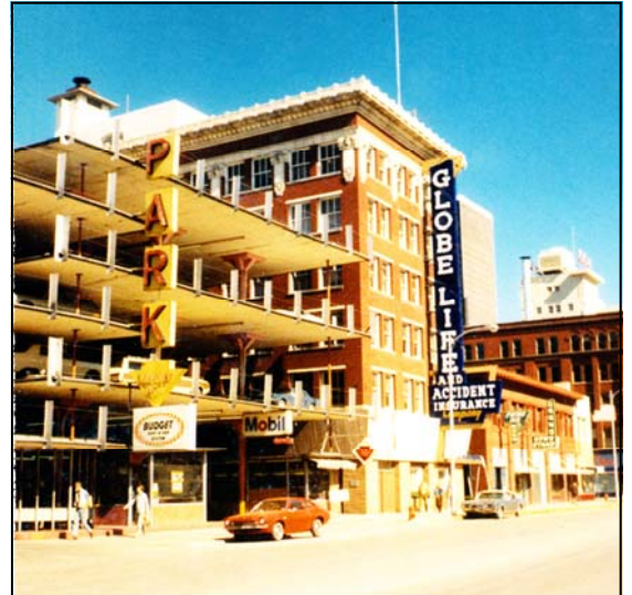
The Globe Life Insurance Building, which we worked on in the 1950s and 1960s. This was formerly the old street car terminal building.
