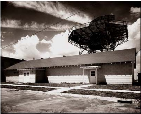
The ARSR-1 radar at FAA in 1959.
